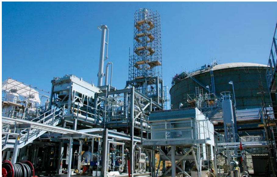
Construction of the $210 million Terasen Gas (Vancouver Island) liquefied natural gas storage facility is nearing completion.
